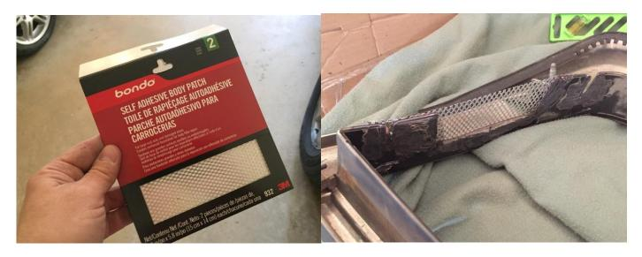
The next step is to use your choice of body filler to cover the backing material in the gaps and any other imperfections on the inside surface.
