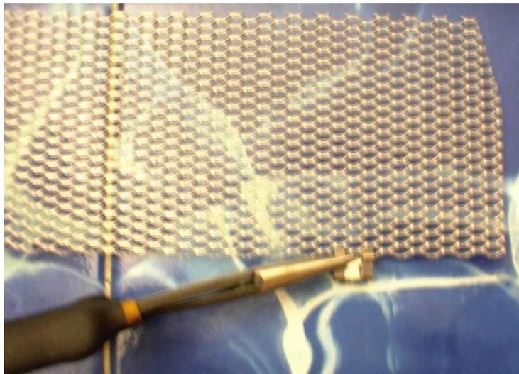
Tighten down the clamping part of the clip to the desired tension. Just take your pliers and close the gap down as far as you want. If you don't tighten them down enough, they will not hold and if you tighten them too much it will be hard to install.
